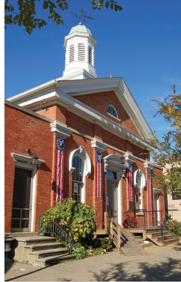
resides on top of the roof today.
