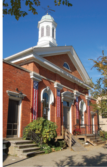
resides on top of the roof today.
